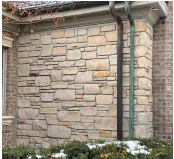
Brushed Grout Example
