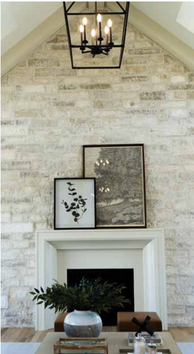
Over Grout Example
